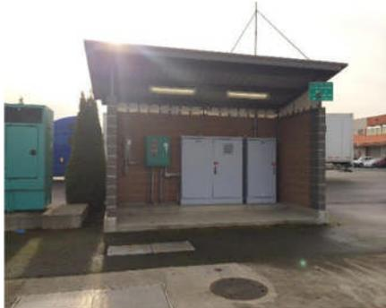
**Improvement:** Revise the control systems at PS-1, PS-5, and PS-6 so that both the emergency power generators and pumps start automatically during a power failure event.
