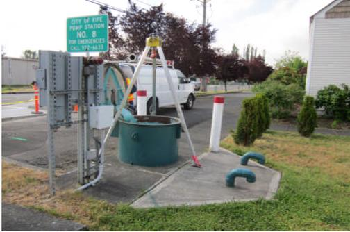
Pump Station 8, located at 6112 20<sup>th</sup> Street East, was constructed more than 20 years ago, was upgraded approximately 7 years ago and serves a mixture of industrial, commercial, and high density residential. This wetwell/drywell type lift station has two pumps, each with a design capacity of 1,200 gpm at 36 feet of discharge head. This station has a 14-inch ductile iron force main that transitions to an 14-inch HDPE. This station has a portable generator converter for standby power.
